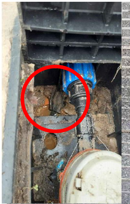
Fraude comercial By pass medidor con Fuga
